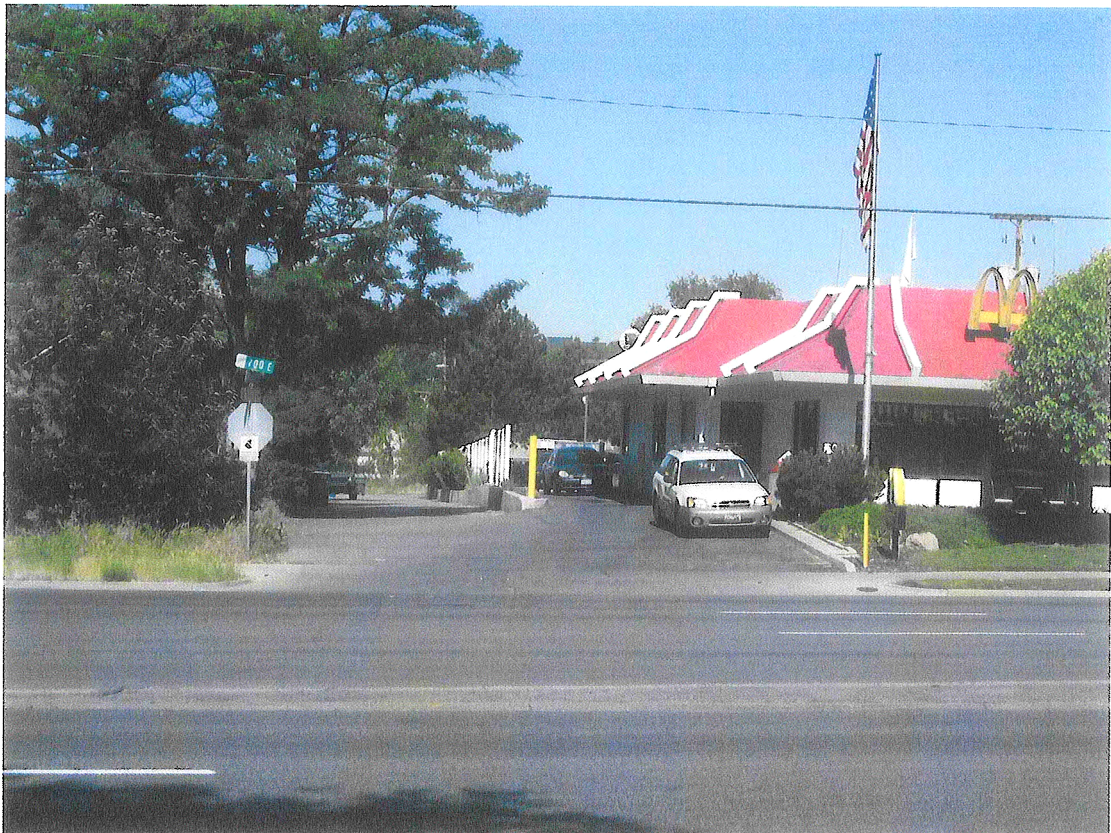
Entrance to Markea Avenue
