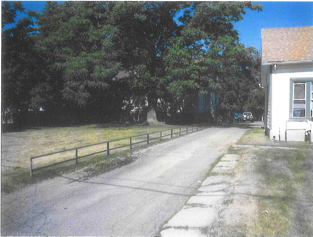
View from 700 East. This driveway will be removed. The house beyond the tree is the six-plex that will remain.
