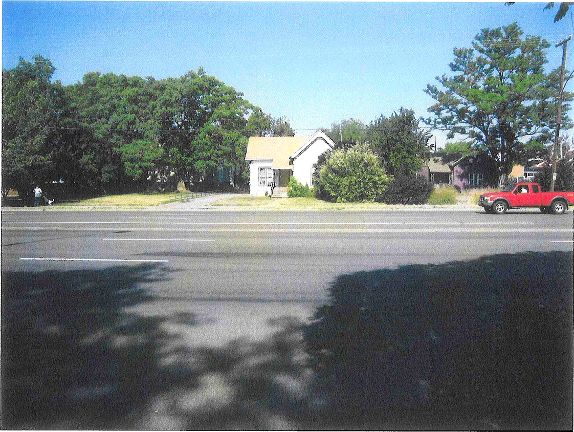
700 East (entrance to Markea Avenue on the far right.) These two structures will be demolished.
